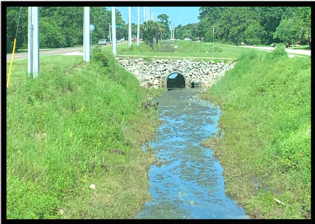
Photo 12: Representative of ditch north of Malabar Road
