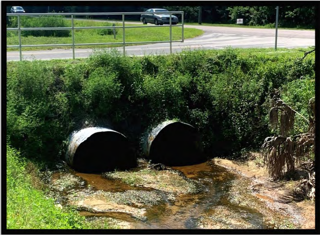
Photo 11: Representative of ditch north of Malabar Road
